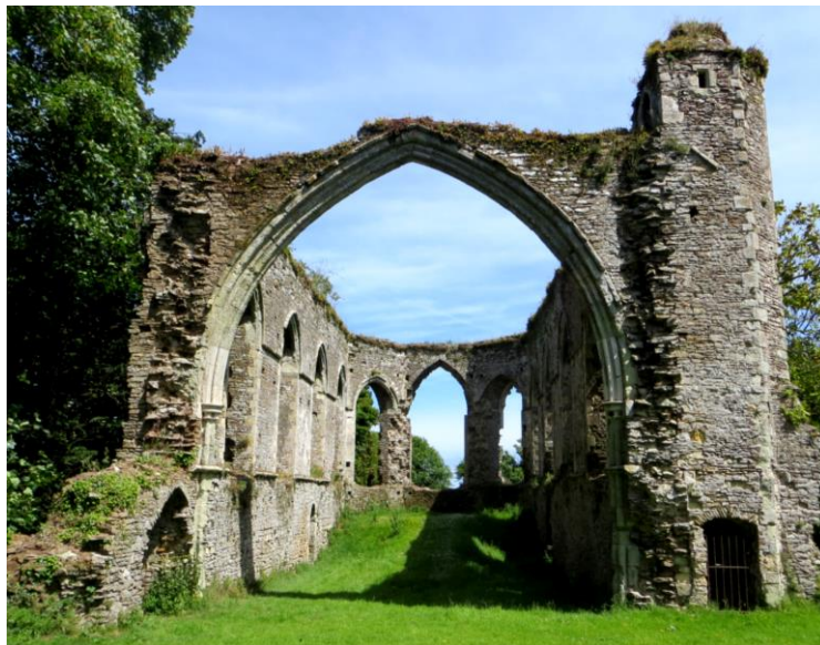
The Chancel of Greyfriars (Franciscan) Priory, Winchelsea (Photos © Keith Foord)
